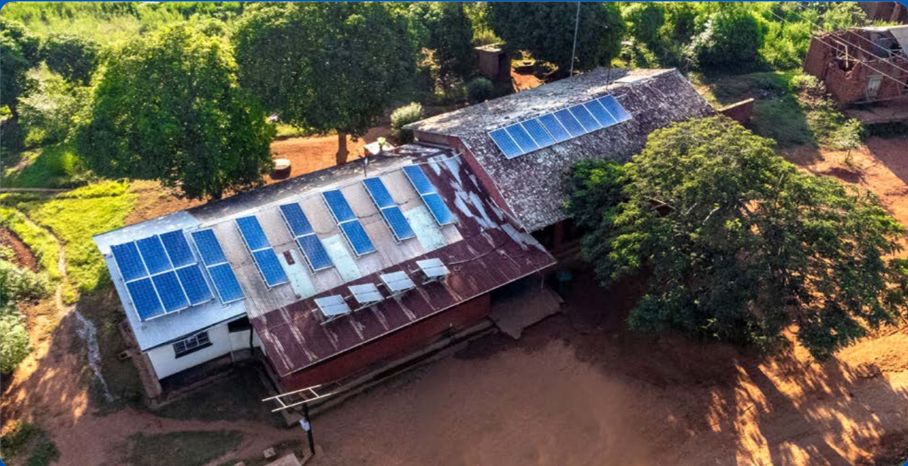
Solar pumped water for district clinic, Thyolo
