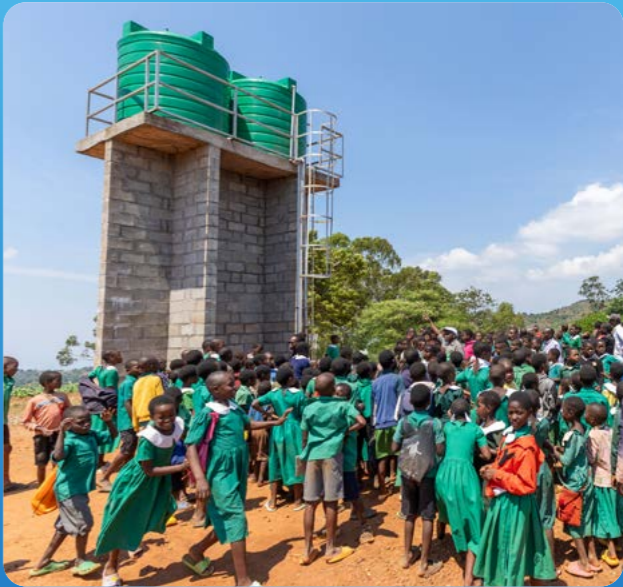
Solar pump storage tanks, Chikwawa Secondary School
