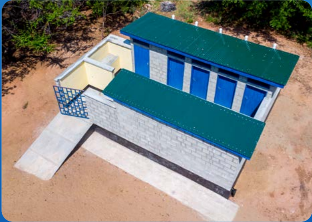
Toilet block, Chikwawa Secondary School
